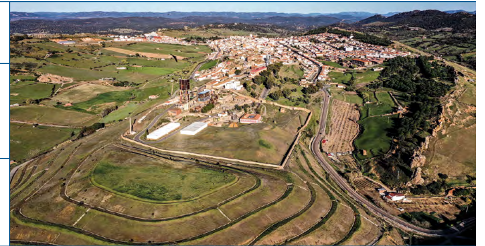
General view of the town of Almadén, Spain, in the foreground are the mercury mining facilities located to the west of the town and in which the main shaft and their metallurgical fence stand out.
